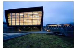
sports facilities Lissfeld Linz 2010
