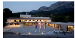
community centre Steinbach am Attersee 2012
