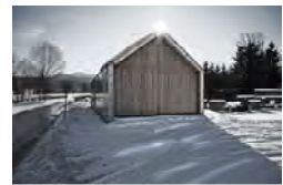
Small hydro power plant Fuschler Ache Thalgau 2011
