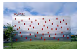
Nave Wallner Scheiffling 2005
